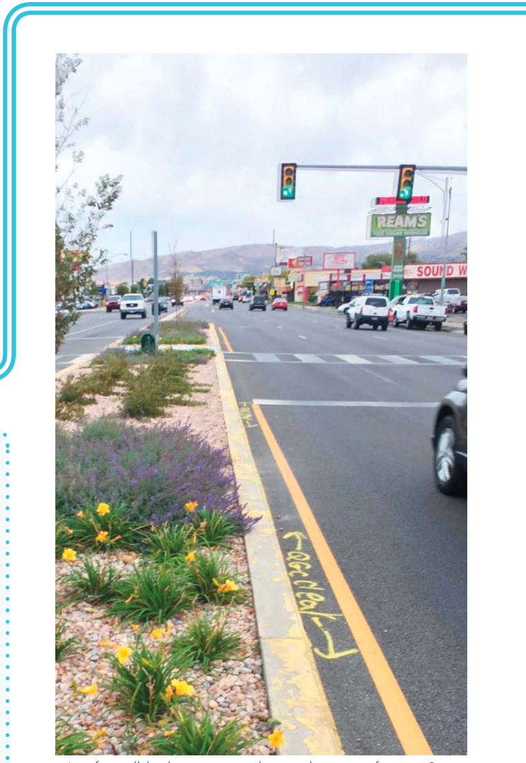
A safe midblock crossing with a pedestrian refuge at State Street and Sunset Ave.
