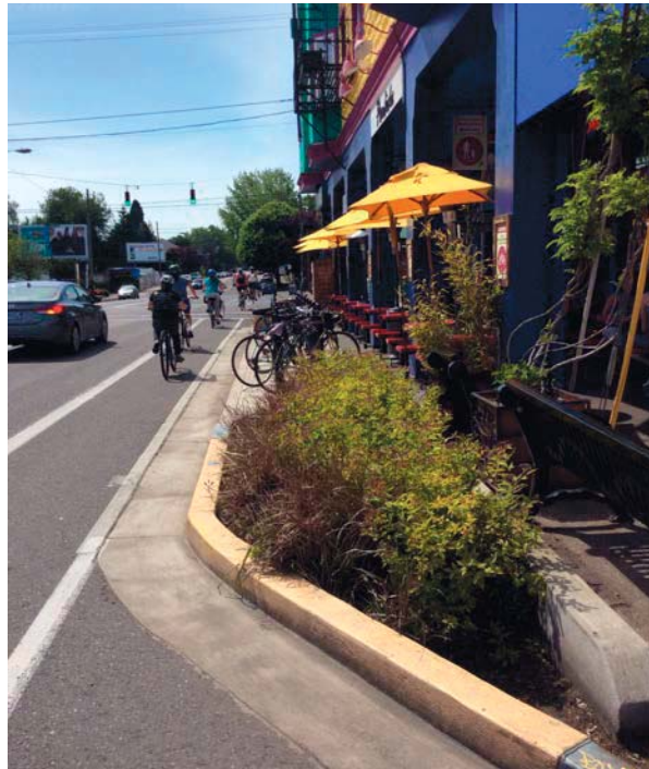
Storm water facility and bike parking space
