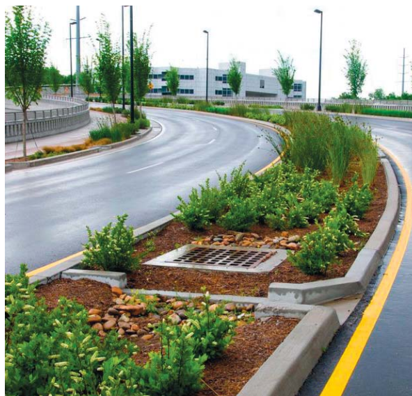
Planted median with integrated storm water infrastructure
