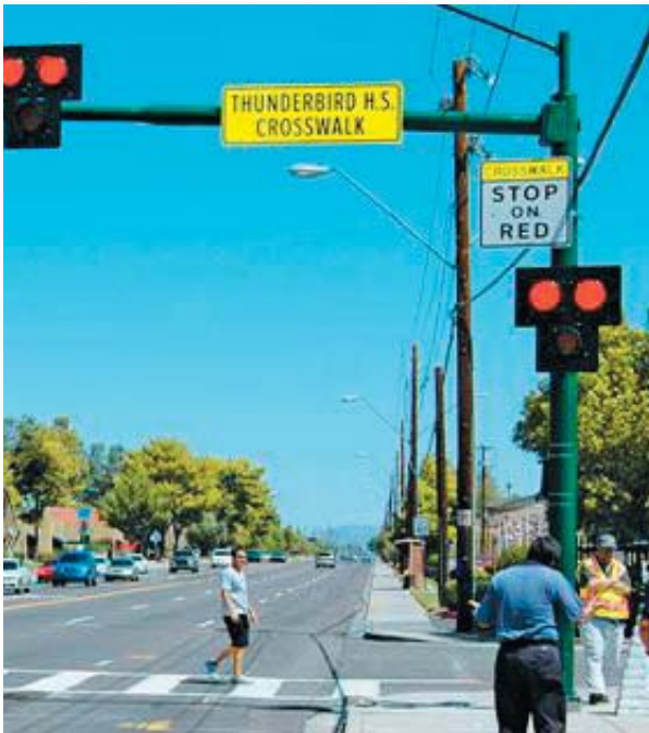
HAWK Beacon pedestrian crossing signal
