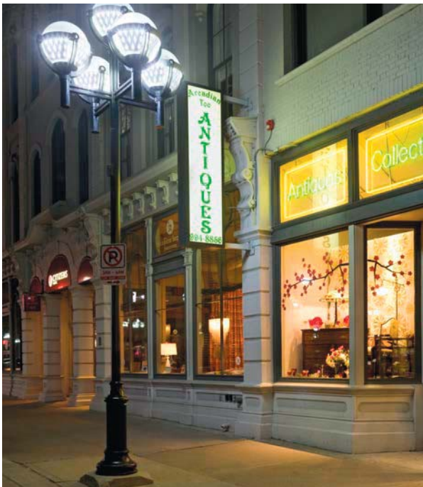
A building with high ground floor transparency
