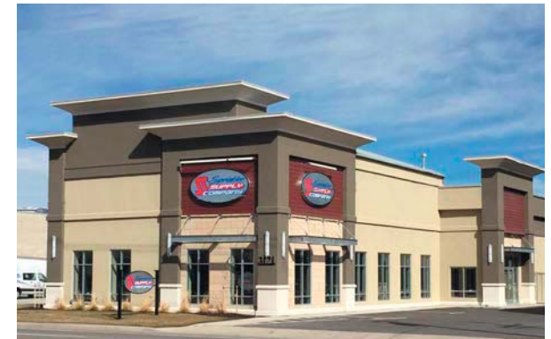
Sprinkler Supply Building at 300 W
