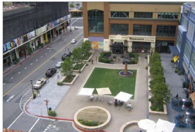
Parks and Plazas should be explored along the State Street corridor. Small plazas can be integrated into urban destinations such as this one.
